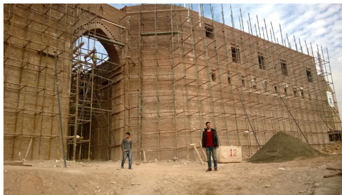
Figure 29: Rebuilding the original Gate in 2013-2014
