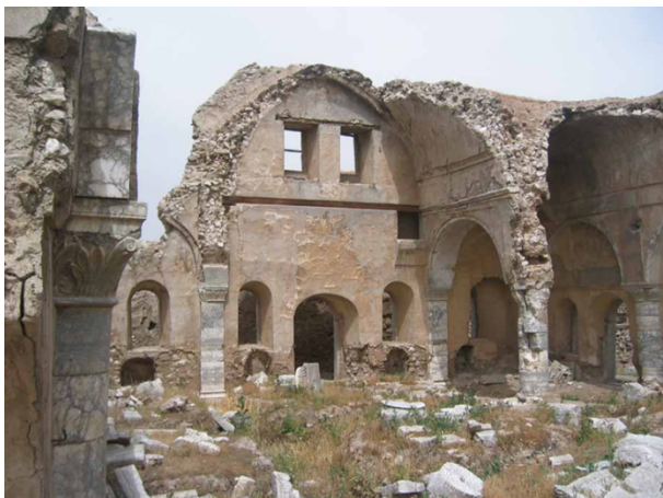
Figure 18: The citadel's buildings after their destructions
