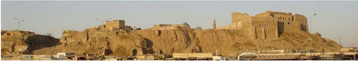
Figure 19: View of the Kirkuk citadel after the destruction
