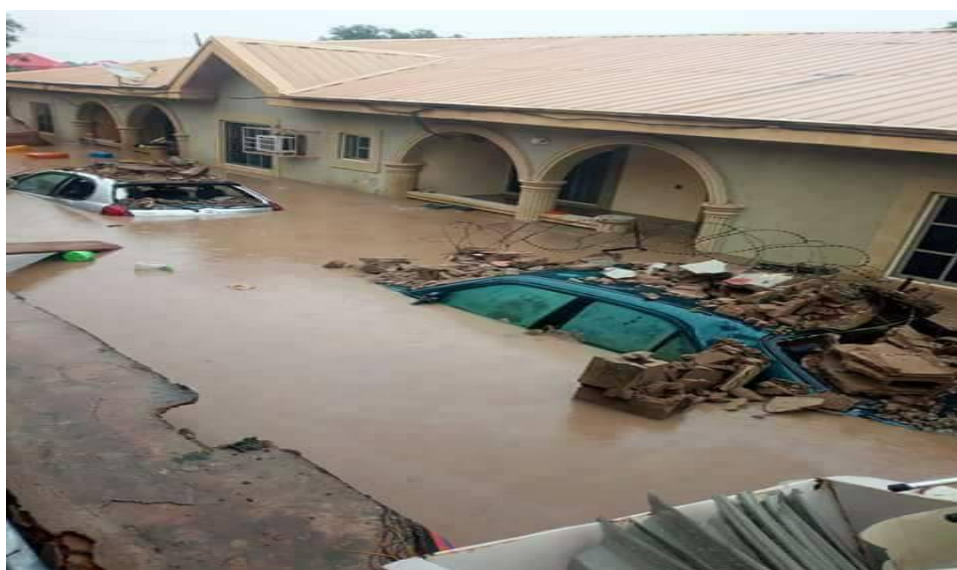
Fig. 2: Flooding causing drowning of cars and houses.
