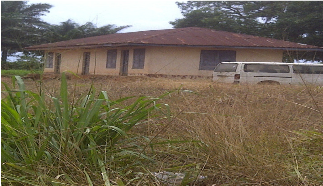
Figure 4: The Primary Health Centre in the community appears unused as it is overgrown with weeds
