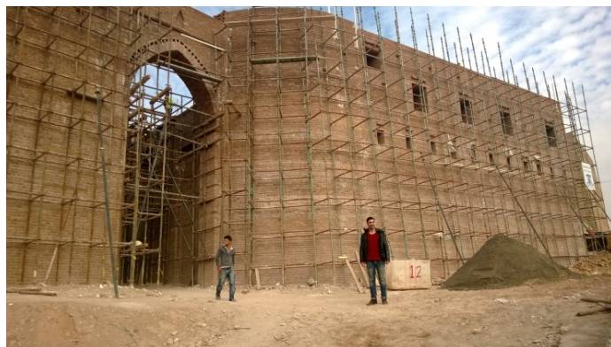
Figure 29: Rebuilding the original Gate in 2013-2014
