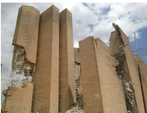
Figure 28: Demolishing the Gate in 2013 Photo: Noor Nooraddin & Osama Nooraddin
