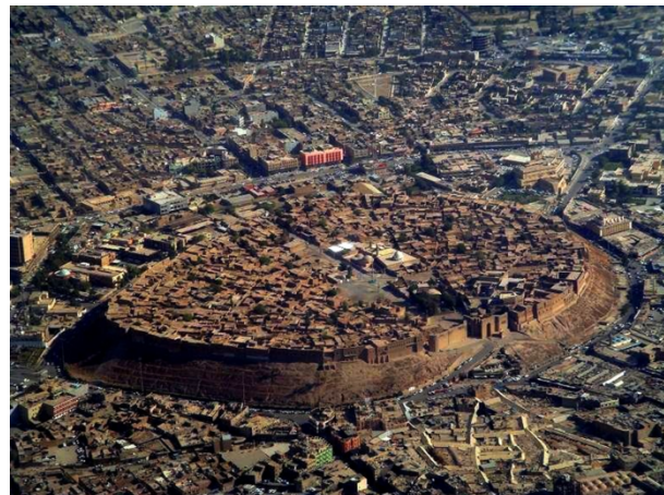
Figure 23: Erbil Citadel 1985: Building a new gate
