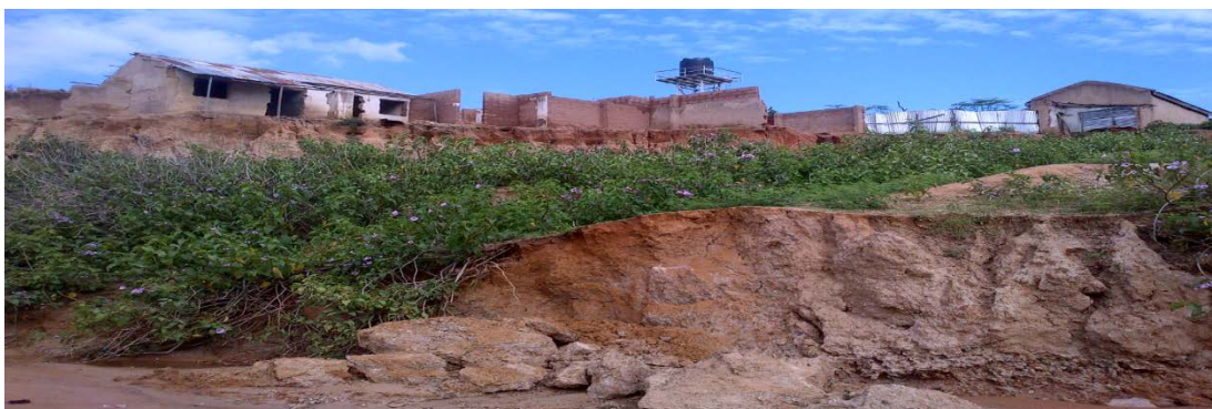
Plate IV: Uncontrolled gully Gully erosion (Arawa, Shamaki ward N10°18'37.8 11 E11°10'43.5 11 )
