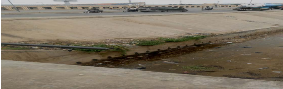
Plate I: Engineering control measure in Pantami ward (stadium) (N 10°16'30.1", E 011°10'02.5)
