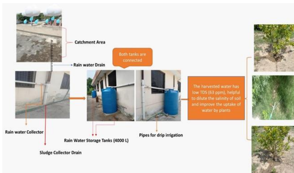
Figure 5: Installed Rain Water Harvesting System in WQL PCRWR-Sahiwal
