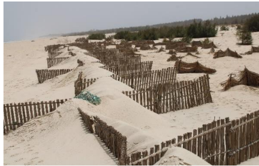
Figure 9: Result of the installation of typhavelles: return of vegetation [2]
