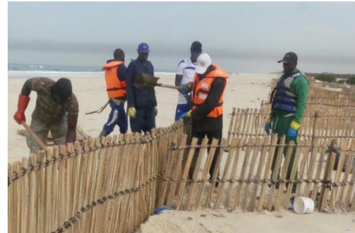
Figure 4: Typha australis typha fences [2] Figure 5: Installation of australis fences [2]
