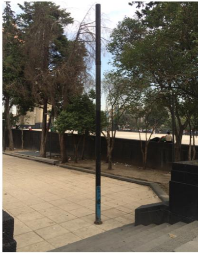
Figure 1: An old steel casing, part of a water well, exposed due to the consolidation of the subsoil
