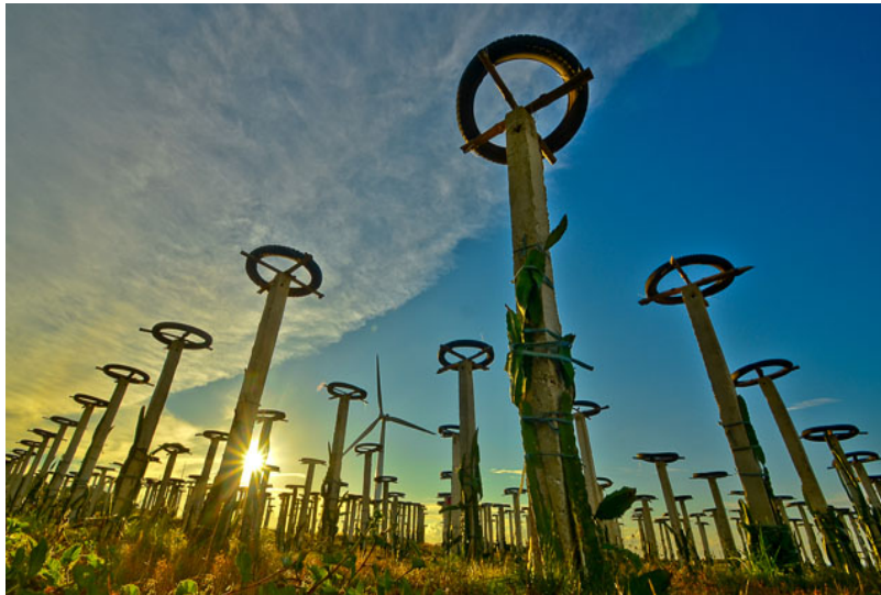
Figure 7: Head cadre of concrete pillar
