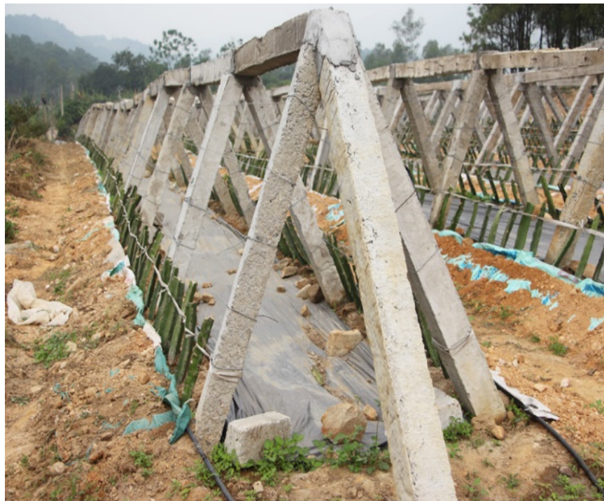
Figure 10: Concrete support cadre
