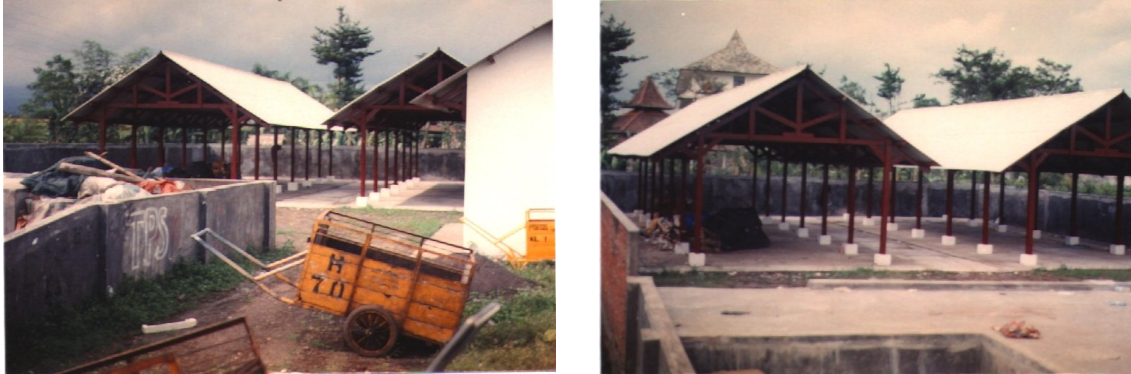
Figure 4: The newly buildings for processing the garbage in TPS RW-08 (Pictures taken during site exploration in March 11-12, 2000)
